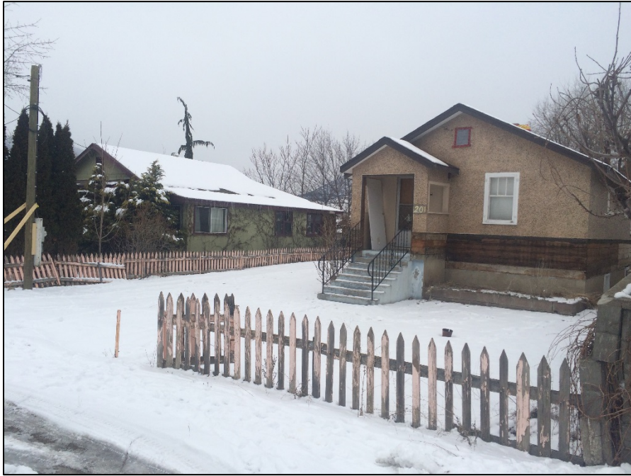
Figure 6: South View showing proximity to west neighbour
